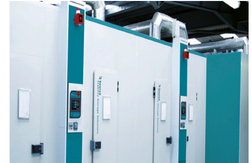
SourceBio Stability Storage service facility
